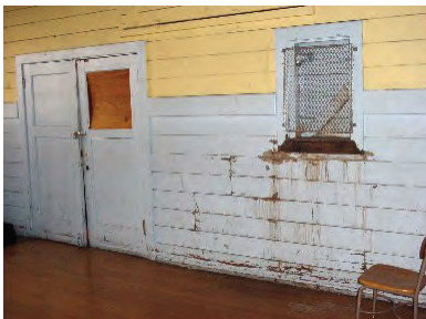
Gym, before renovation
